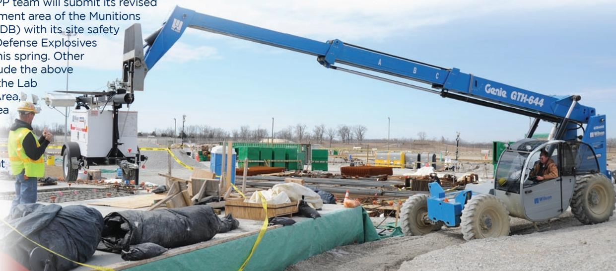
Bechtel Parsons Blue Grass staff direct an overhead crane to position a generator on the foundation for the Munitions Demilitarization Building. The generator will supply additional power for temporary lighting which will be used to illuminate early morning concrete placements.
