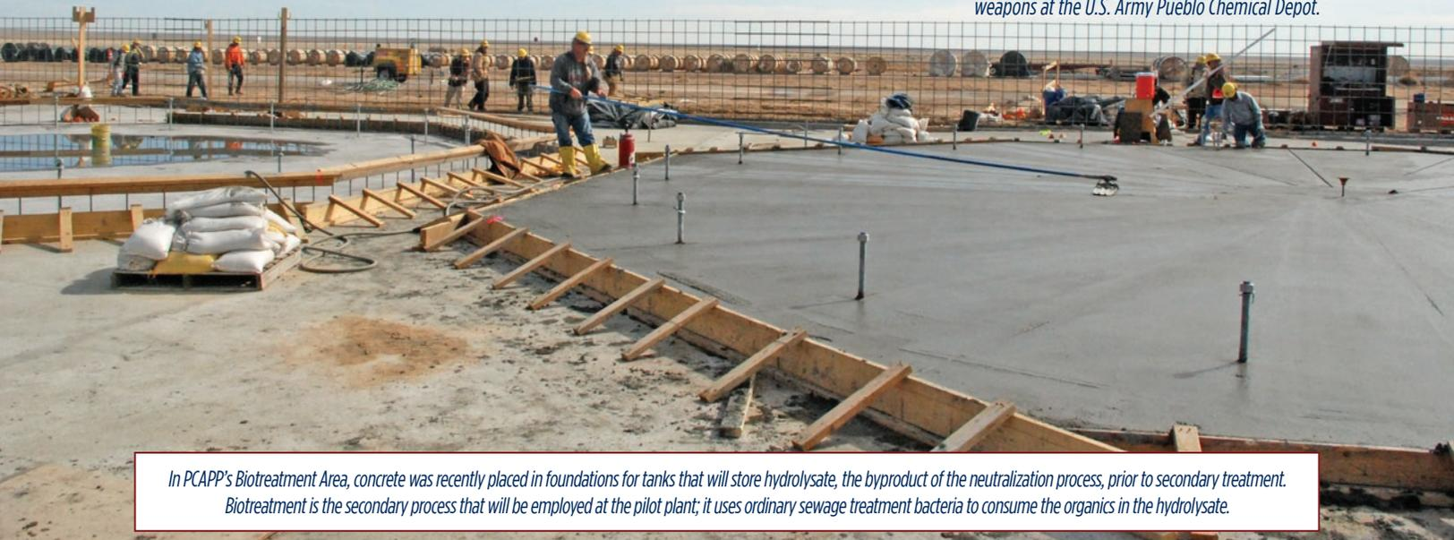
*In PCAPP's Biotreatment Area, concrete was recently placed in foundations for tanks that will store hydrolysate, the byproduct of the neutralization process, prior to secondary treatment. Biotreatment is the secondary process that will be employed at the pilot plant; it uses ordinary sewage treatment bacteria to consume the organics in the hydrolysate.*
