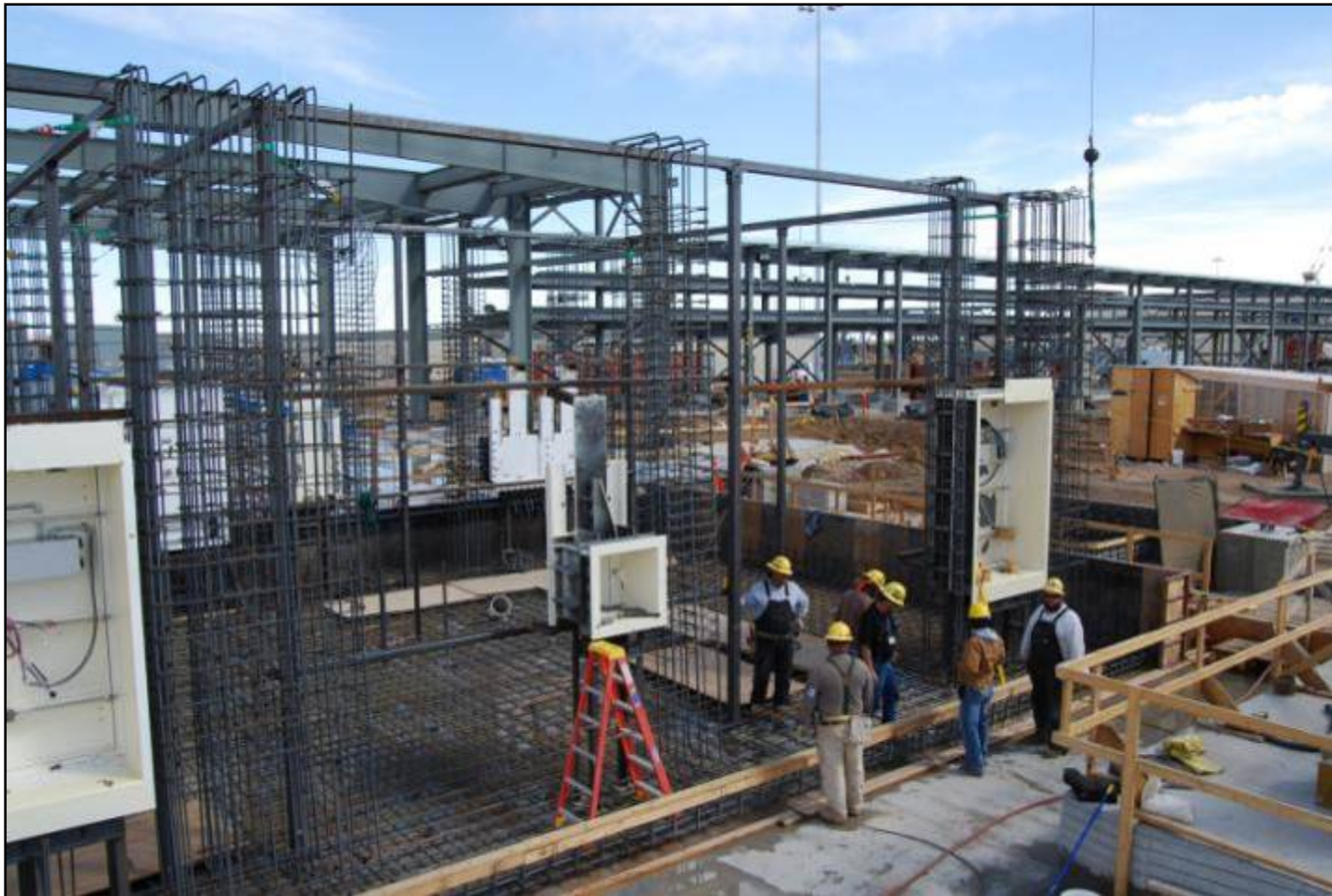
Structural steel is being erected for the Explosive Containment Rooms.
