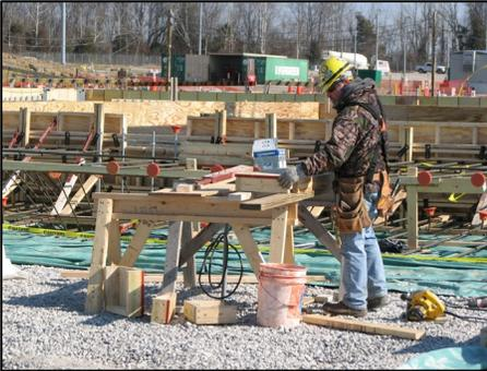
**Photo 1 (worker constructing wood framing):** A Bechtel Parsons construction worker builds framing for the first major concrete placement for the foundation of the Munitions Demilitarization Building at the Blue Grass Chemical Agent-Destruction Pilot Plant.
