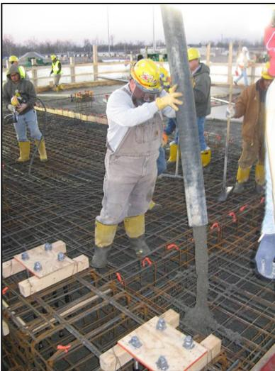
**Photo 3 (worker directing concrete spout):** A Bechtel Parsons construction worker spreads concrete during the first major concrete placement for the Munitions Demilitarization Building at the Blue Grass Chemical Agent Destruction Pilot Plant.
