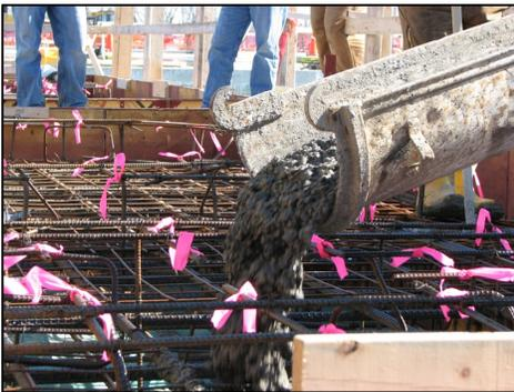
**Photo 2 (concrete flowing from chute):** Concrete flows from a chute into a wire-reinforced form as part of the first major concrete placement for the foundation of the Munitions Demilitarization Building at the Blue Grass Chemical Agent-Destruction Pilot Plant.
