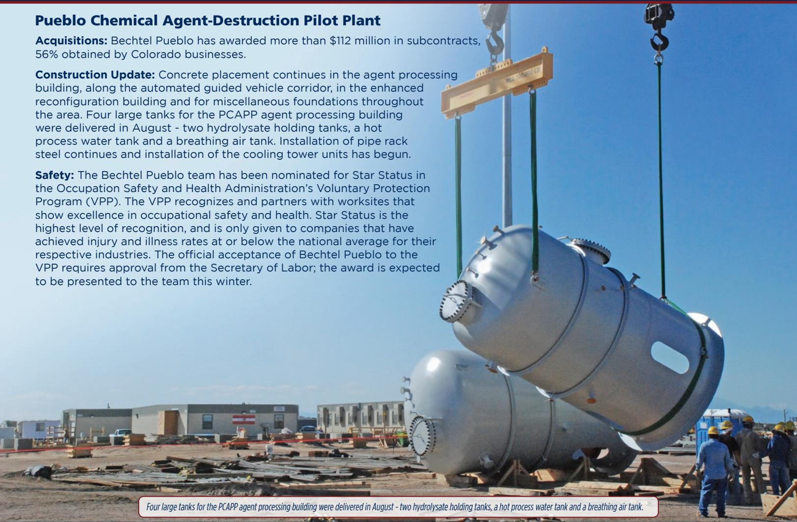
Four large tanks for the PCAPP agent processing building were delivered in August - two hydrolysate holding tanks, a hot process water tank and a breathing air tank.
