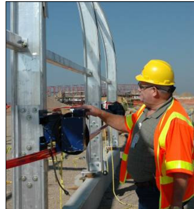
Safety Manager Terry Wells checks equipment that will be used to stretch fabric over Access Control Point structures.
