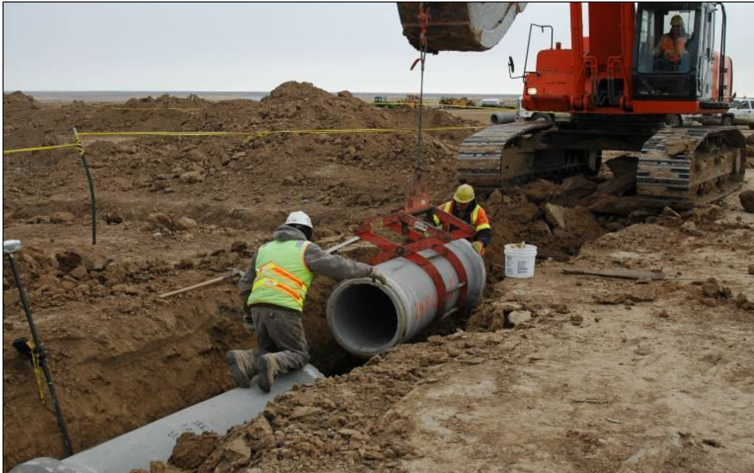
Workers from RBK Construction place culverts
