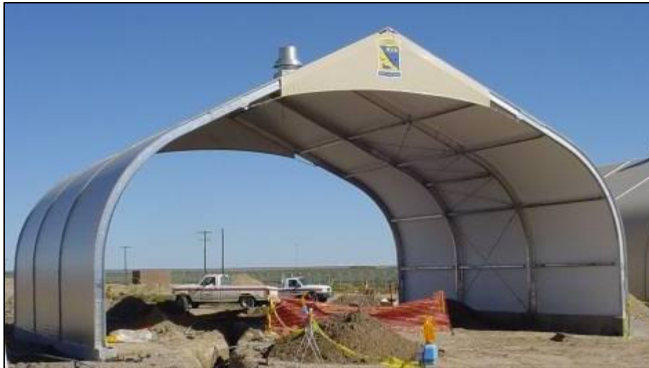
Vehicle Inspection Station
