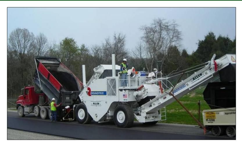
Laying final asphalt surface on the nearly-complete site access road.
