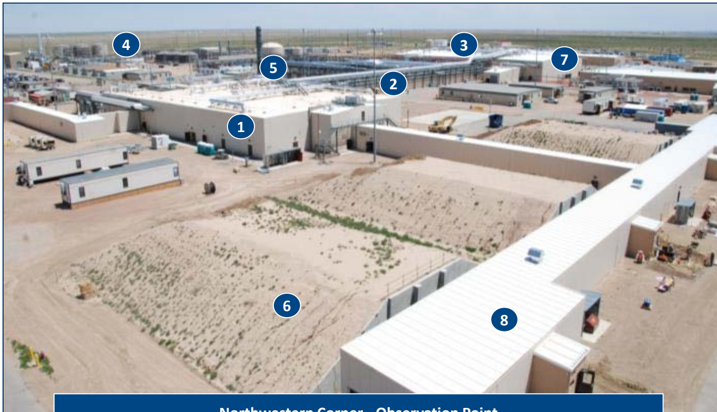
Northwestern Corner - Observation Point
