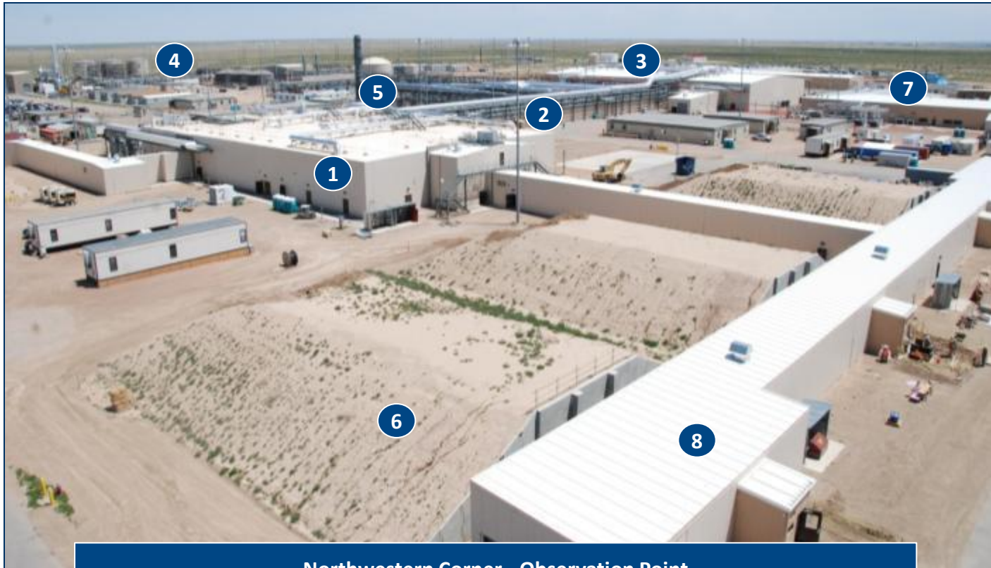
Northwestern Corner - Observation Point
