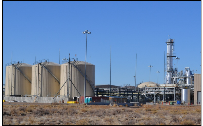
The Brine Reduction System is the final stage of the PCAPP biotreatment process. A secondary waste of dried salt cakes will be shipped off-site to a permitted hazardous waste facility.
