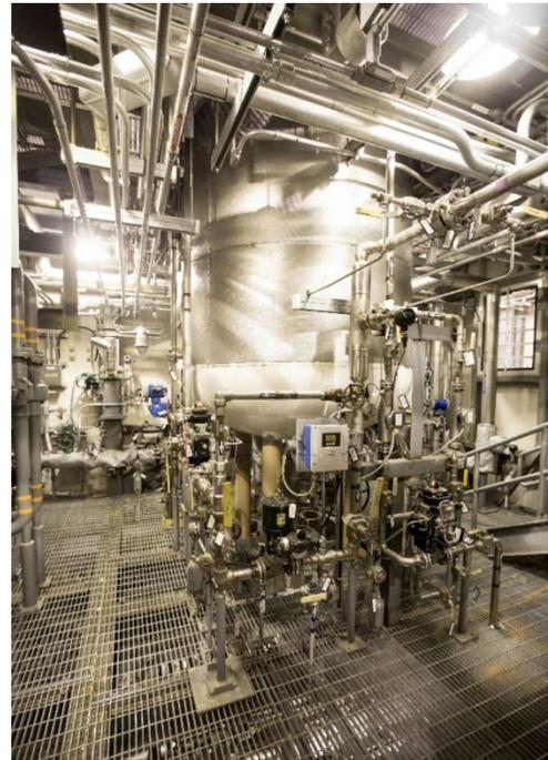
*An Agent Neutralization Reactor stands in the Munitions Demilitarization Building at the Blue Grass Chemical Agent-Destruction Pilot Plant. Nerve agent drained from rockets and projectiles was pumped to this reactor and mixed with hot water and sodium hydroxide to neutralize the agent. The resulting product was known as hydrolysate.*
