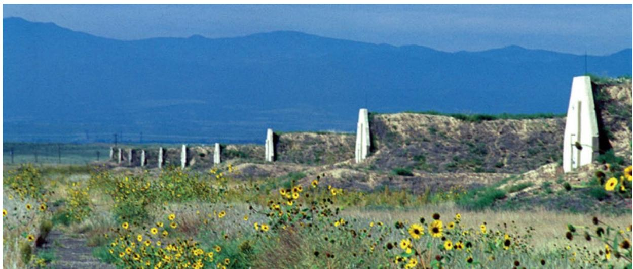
*These specially designed earth-covered magazines, commonly referred to as storage igloos or bunkers are located on the highly secure U.S. Army Pueblo Chemical Depot where all Department of Defense and Army safety and security regulations are followed.*
