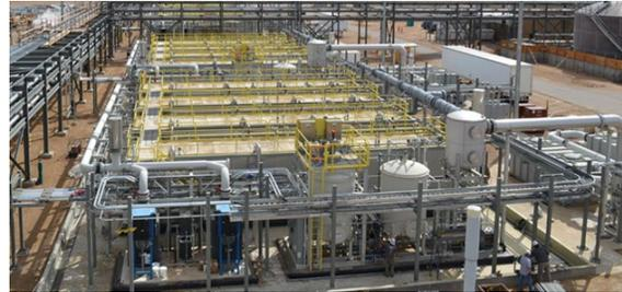
*The Immobilized Cell Bioreactors located on the PCAPP site use common microbes to treat hydrolysate.*
