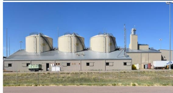
*The Brine Reduction System is the final stage of the PCAPP biotreatment process. A secondary waste of dried salt cakes are shipped off-site to a permitted hazardous waste disposal facility.*
