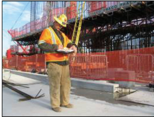
Photo 2: Inspection of equipment
