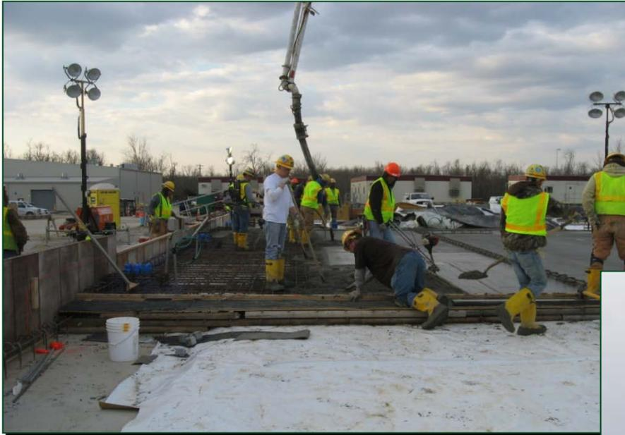
BGCAPP craft workers completed another SCWO concrete foundation placement (at left); and continued reinforcing steel installation to prepare for more concrete placements.
