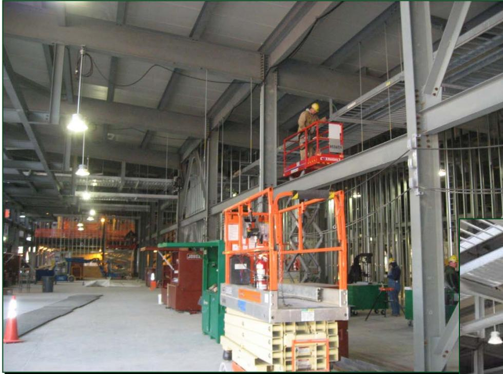
BGCAPP craft workers' efforts to safely install electrical cable tray and metal wall studs are taking shape within the CSB.
