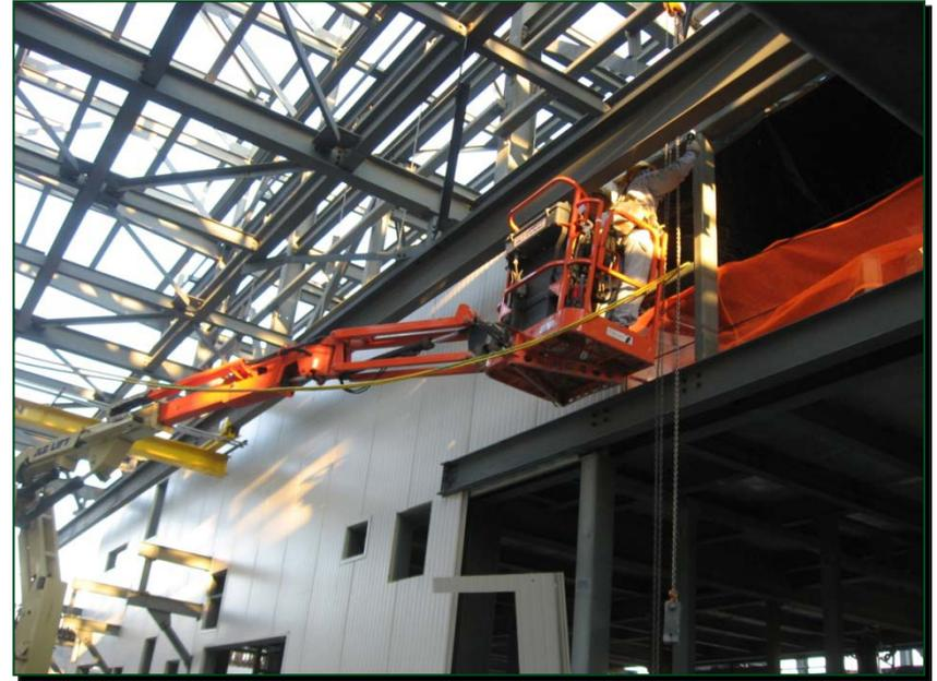
**BGCAPP construction craft workers (above left) make an early morning MDB concrete wall placement. Meanwhile, interior wall panels are being installed (above right) within the MDB. The MDB is where the chemical weapons will be disassembled, explosives removed and the agent neutralized.**
