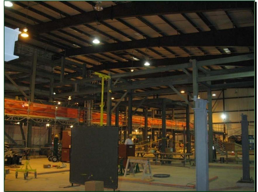
The UB, which will house equipment to produce steam, compressed air, chilled water and hot water for operations, is a hub of indoor activity. BGCAPP craft workers (above left) continued installing support steel and equipment around a trio of placed boilers. At the opposite end of the UB (above right), workers are fitting, installing and welding piping.
