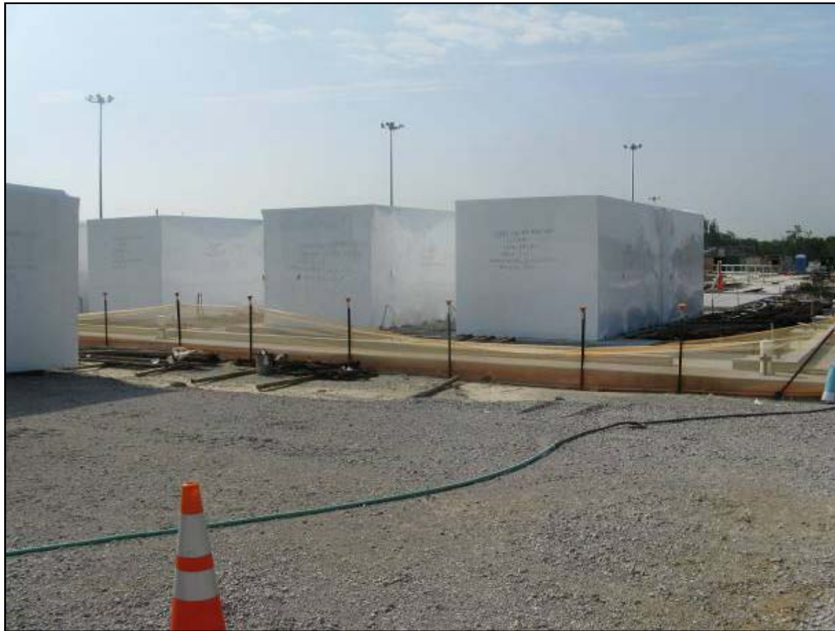
Large air-handling units are positioned for final placement.
