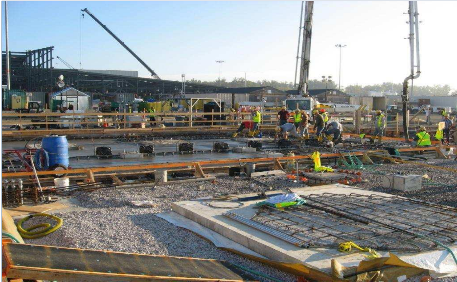
The first concrete slab is being placed for the SCWO Building.
