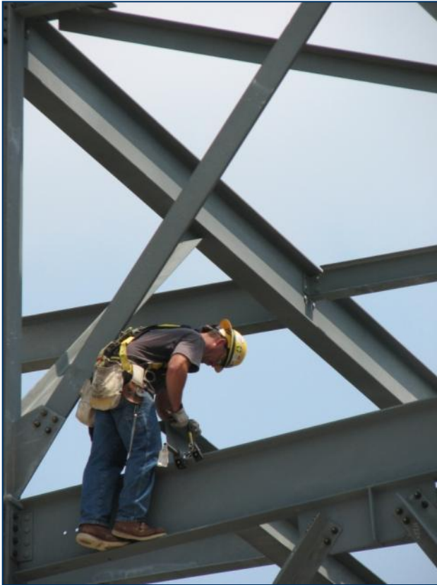
BGCAPP Worker installing structural steel for Control and Support Building.
