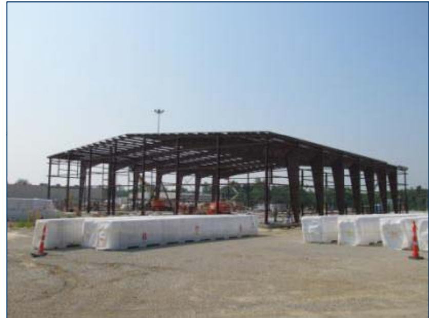
Utility Building is one of several current construction activities.
