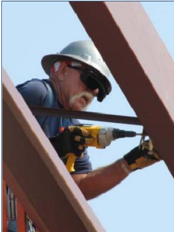
Worker installs structural steel for roof of Utility Building.
