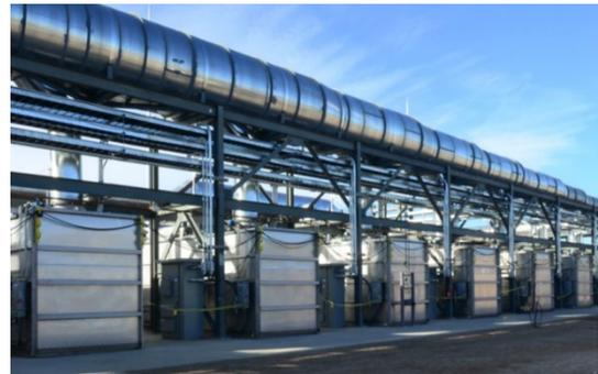
*The Agent Filtration Area consists of eight, plus one standby, one in maintenance filter units (six shown above) that filters the air used in two buildings during the chemical weapons destruction process*
